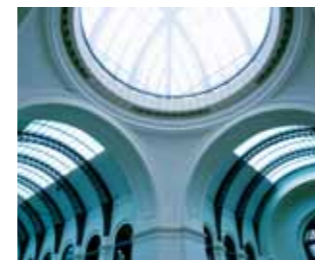
Gare Principale, Dresdes Architecte: Sir Norman Foster, Sir Norman Foster, Foster + Partners, Londres
